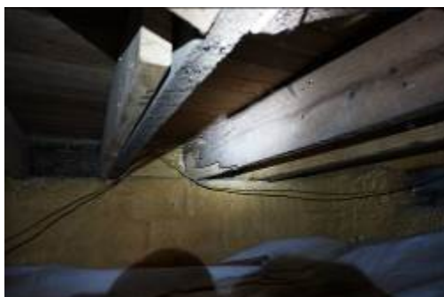
Figure 1-Termite activity in joist
