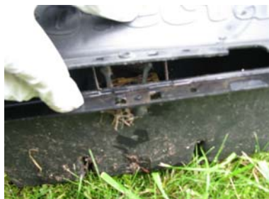
Fig.4 Broken latch NW corner
