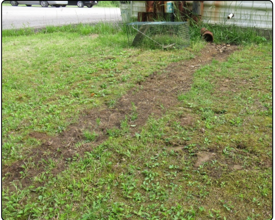
Drain discharge with evidence of run-off (File 83459)
