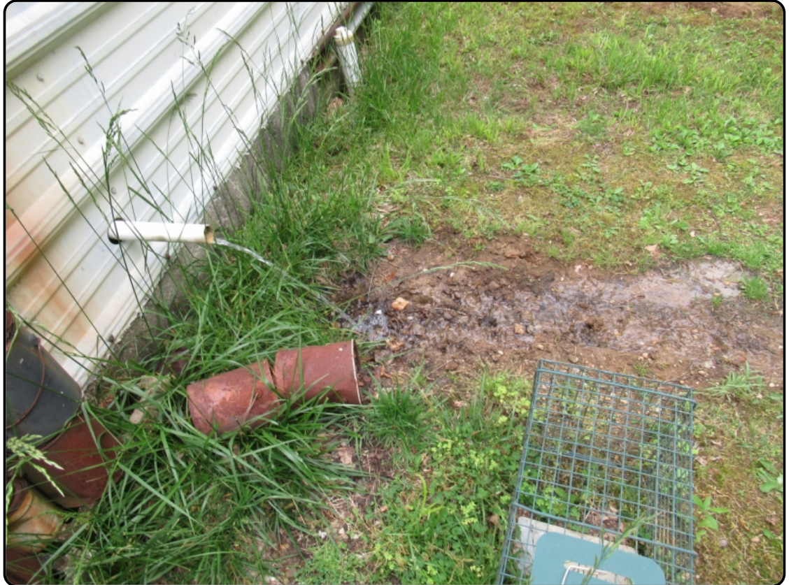
Drain discharge with evidence of run-off (File 83459)
