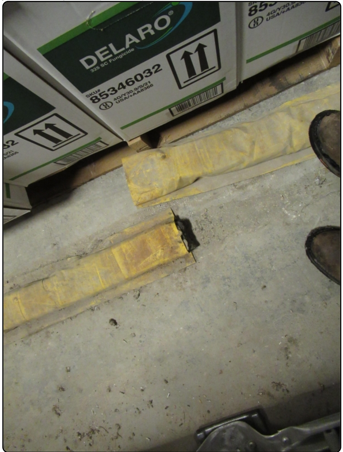
Poly/Foam Wall Separation (File 86963)
